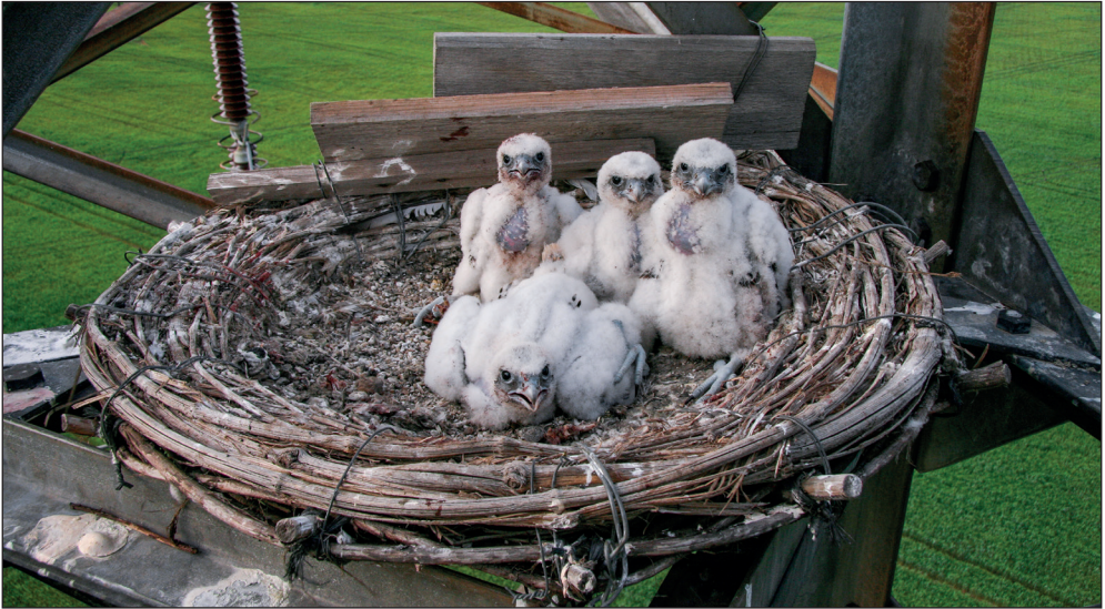
Figure 8. We also installed nest platforms in a few numbers on several transmission line towers, which falcons also like to occupy (ringing, May 2003). Photo: J. Chavko
